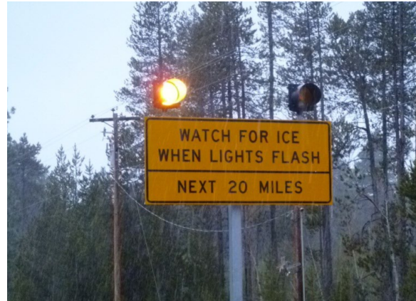
Photo/Image Credit: Kittelson photo on OR 140 illustrating weather warning system.
