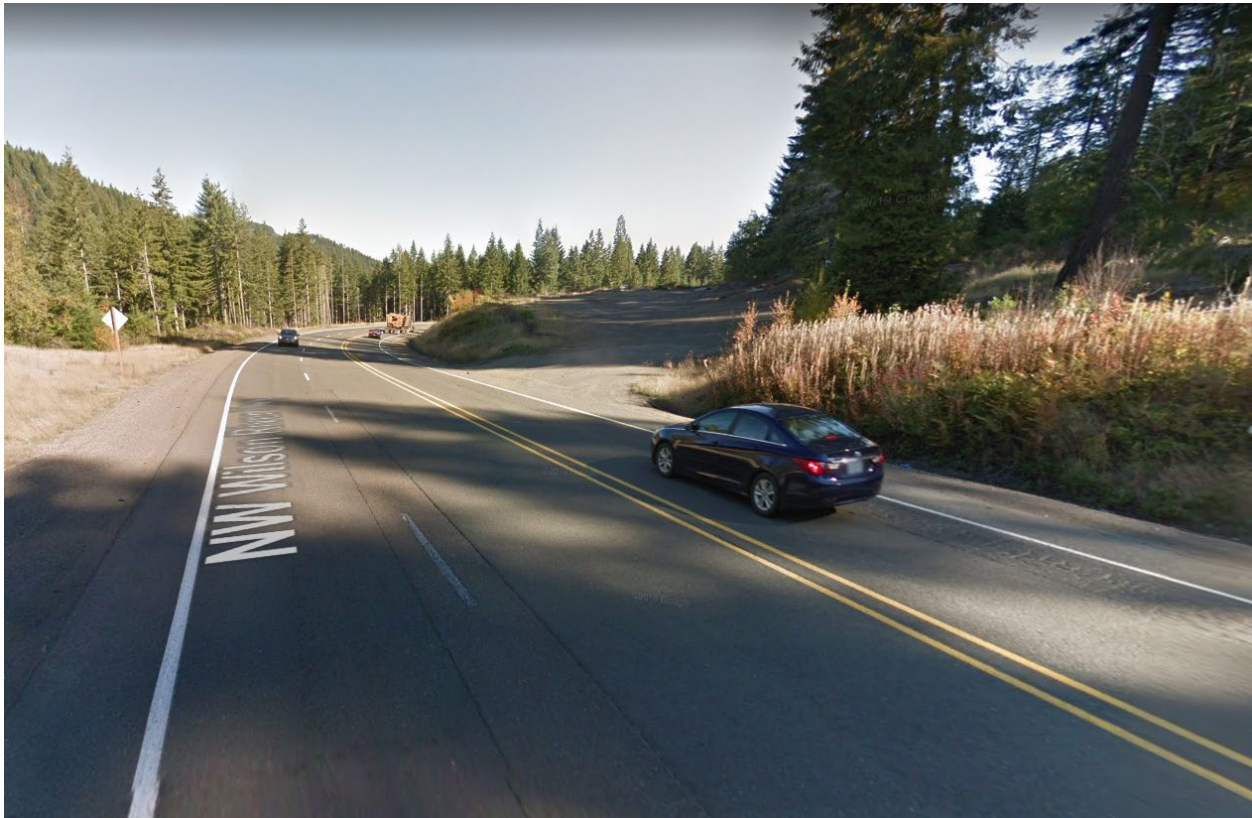
Exhibit 3. Passing Lane with Left-Turning Movements near Merge at M.P. 33.55. (Photo Source: Google Earth Street View).
